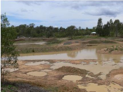
(LEFT) was created many years ago by diverting the flow of a natural watercourse. It has now been upgraded to form a large dam which provides water for the resort. Surplus water flows through a pipe to another dam which contains an island and then flows through another pipe to re-join the original watercourse.
